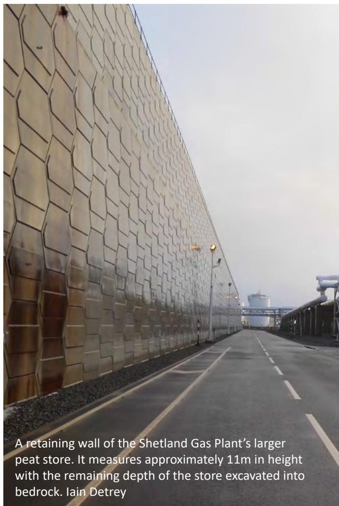
A retaining wall of the Shetland Gas Plant's larger peat store. It measures approximately 11m in height with the remaining depth of the store excavated into bedrock. Iain Detrey
