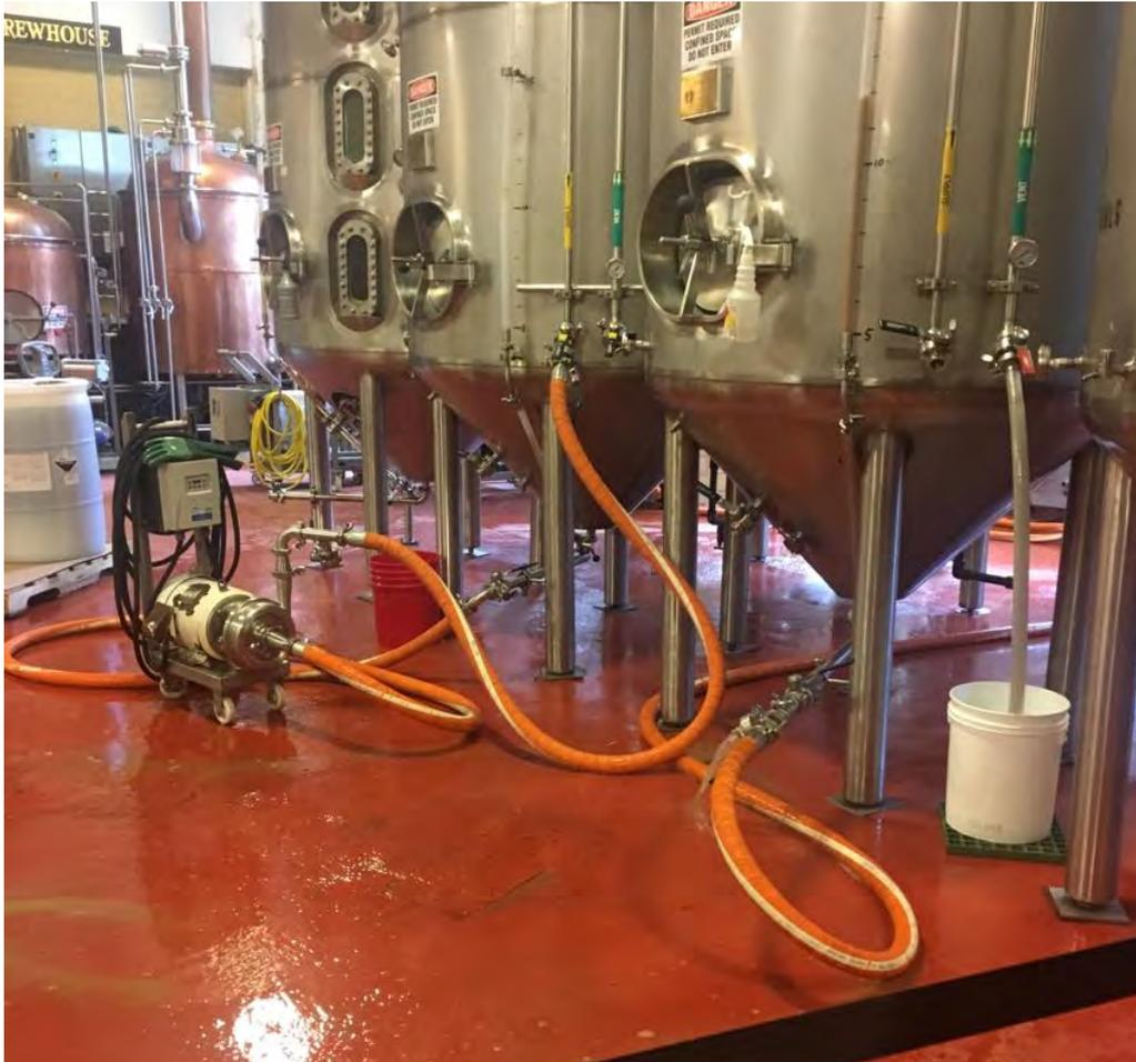
**Figure 15:** Cleaning equipment used on fermentation tanks
